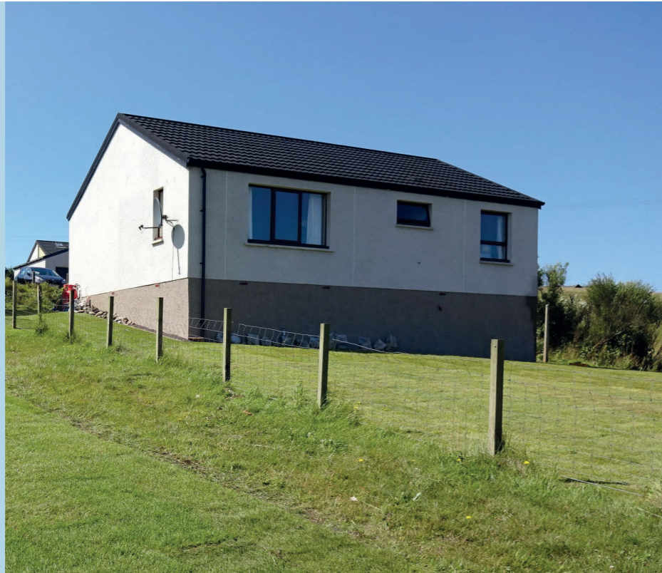
Blockwork replacement - Hillock, Boddam
